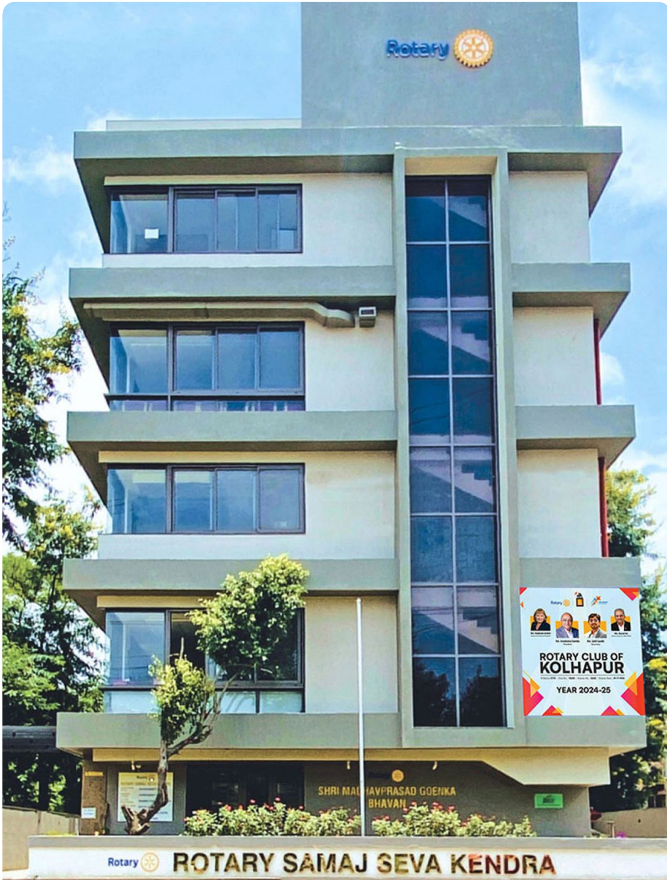
ROTARY CLUB OF KOLHAPUR'S ROTARY SAMAJ SEVA KENDRA BUILDING
